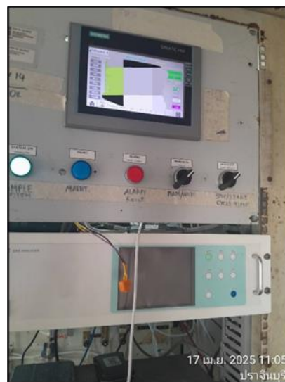
CEMs Recovery Boiler
