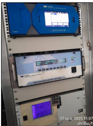
CEMs Power Boiler
